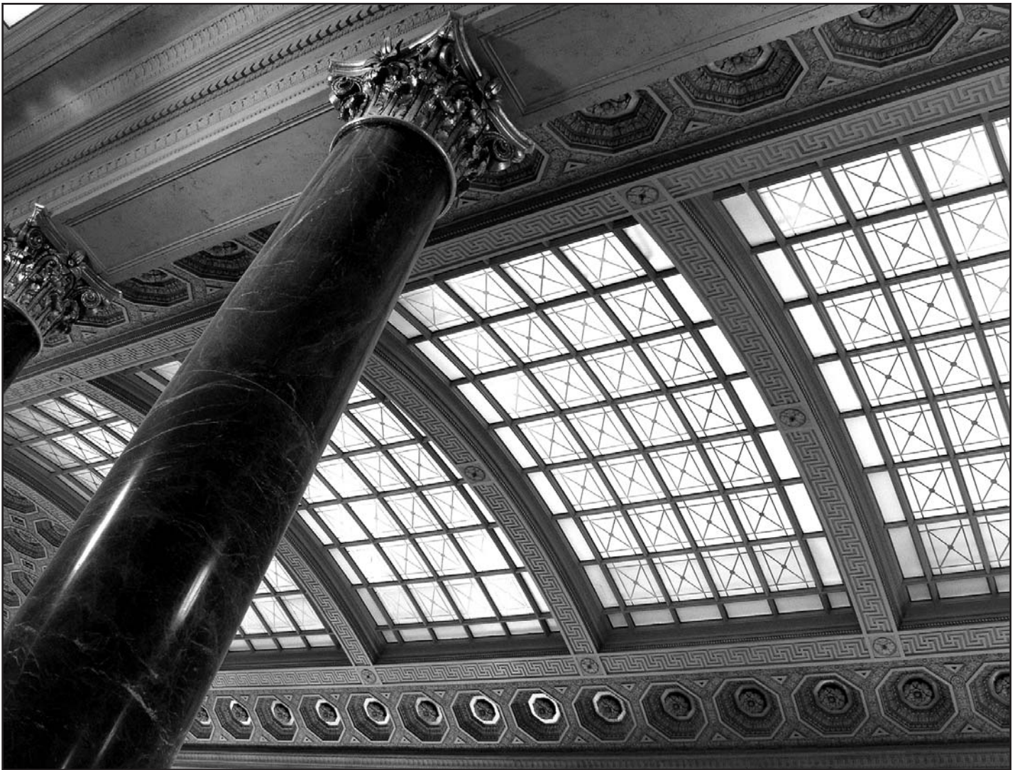
The Conrad Schmitt Studios project at Walter Library was not merely a restoration of the past's glory but an anticipation of the needs of the future. It included mechanisms to allow wiring to be added in the future in anticipation of new technologies and even includes one room rebuilt on a floating steel floor deck to allow easy addition of any cabling or similar elements in an extremely cost-effective manner in the future. Photograph by Dana Wheelock.
