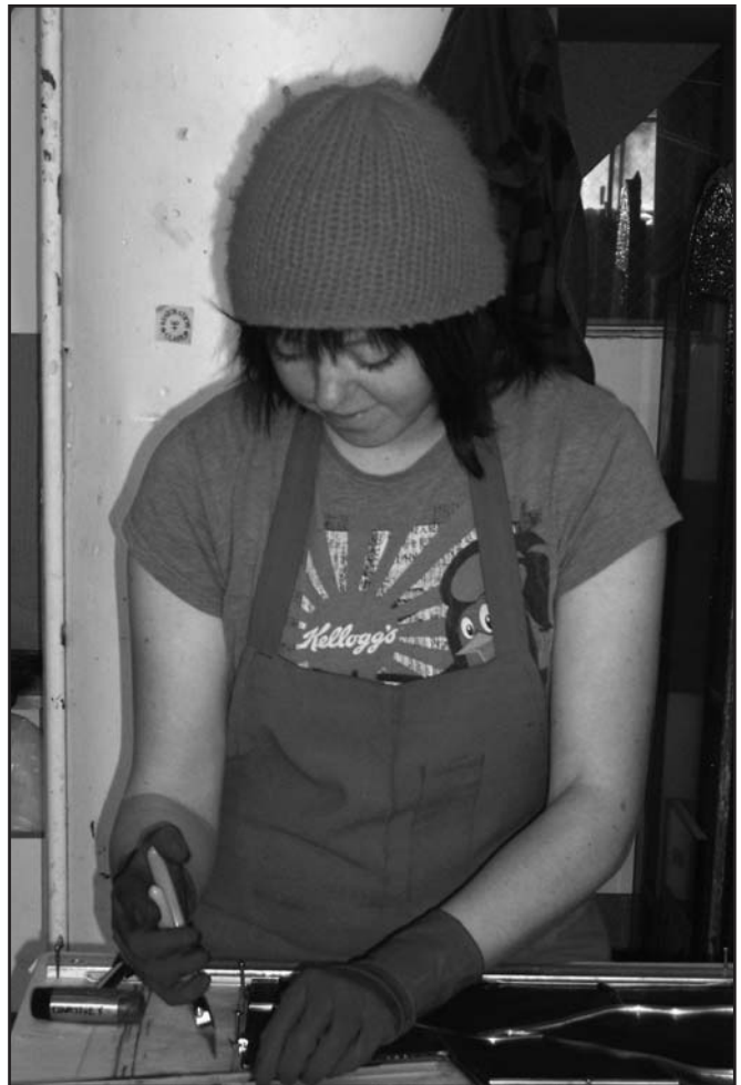
Courtney Dragge releading a St. Luke window panel.
