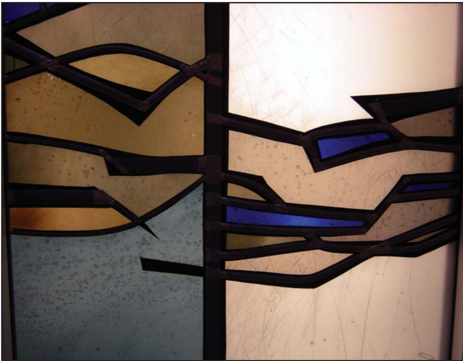
Detail of painting to extend leads and a good example of the “wischen” technique.
