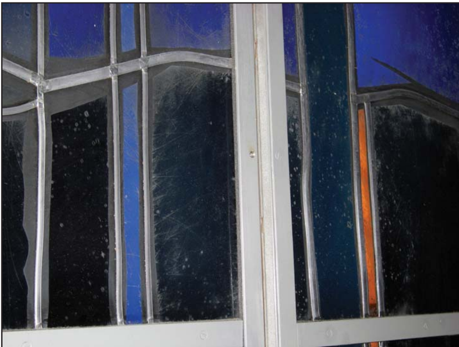
Reflected light view. Note the painted areas that serve as the lead extensions as well as the “wischen” technique.
